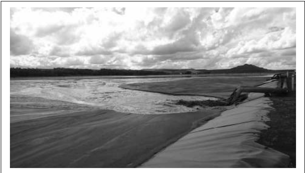
Figure 5: The Tailing Storage Facilities (TSF) of CMOC Brasil (Niobras) in Catalão
