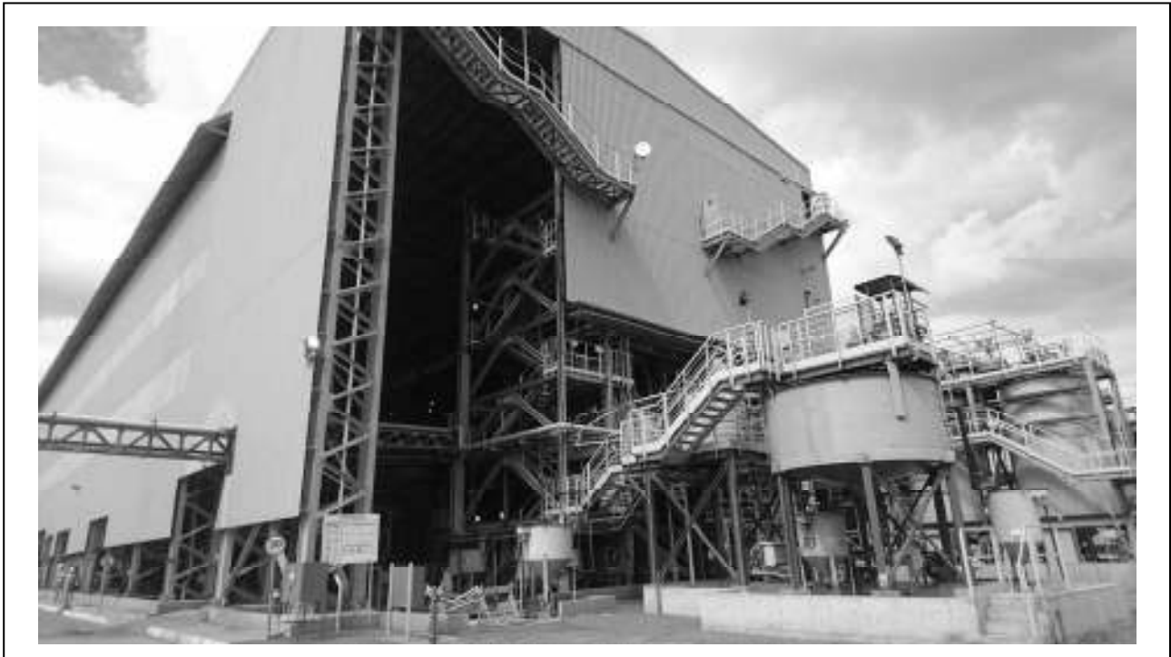
Figure 6: The Boa Vista Fresh Rock (BV FR) Processing Plant of CMOC Brasil (Niobras) in Catalão
