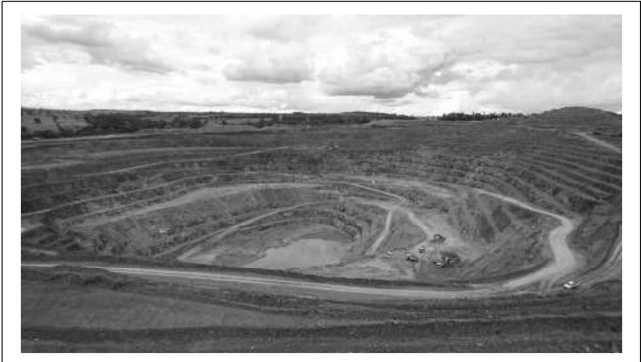
Figure 2: The CMOB Brasil (Niobras) Boa Vista mine close to Catalão, which contains REE bearing minerals
