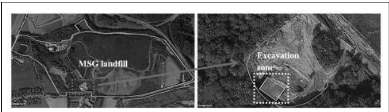
Figure 1: MSG landfill (left) and excavation zone (right) [7].
