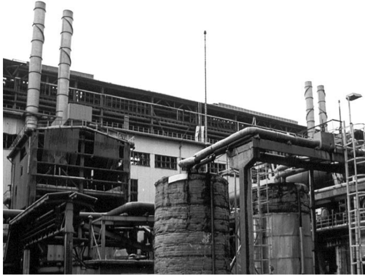
Figure 6: Ferronickel plant in Glogovac, Kosovo
